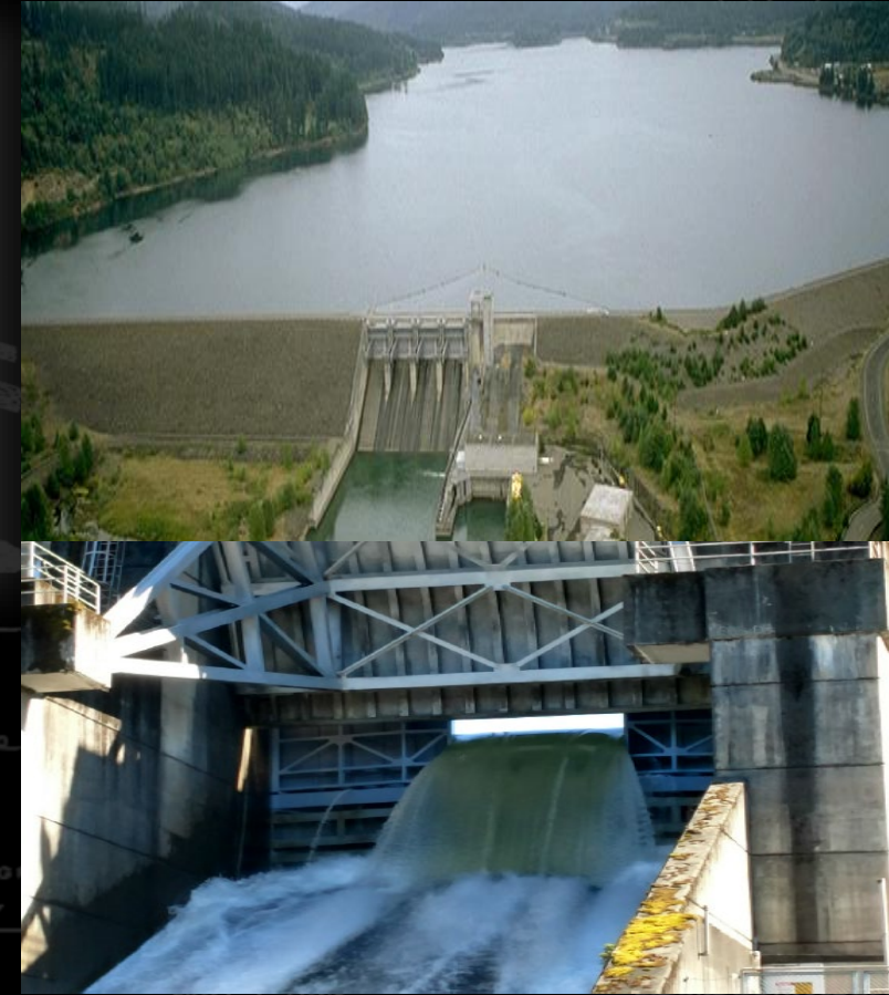
New Spill Weir, Foster Dam (2018)
